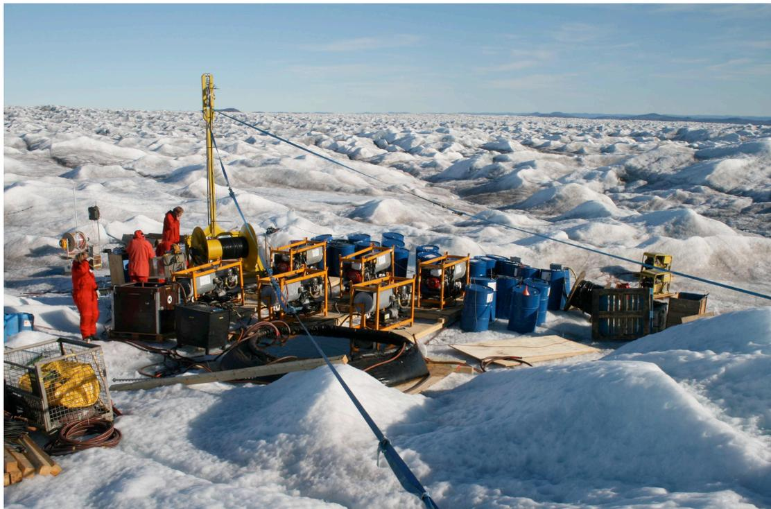
Figure 2. The hot water drill from the AWI in operation at the field site.
